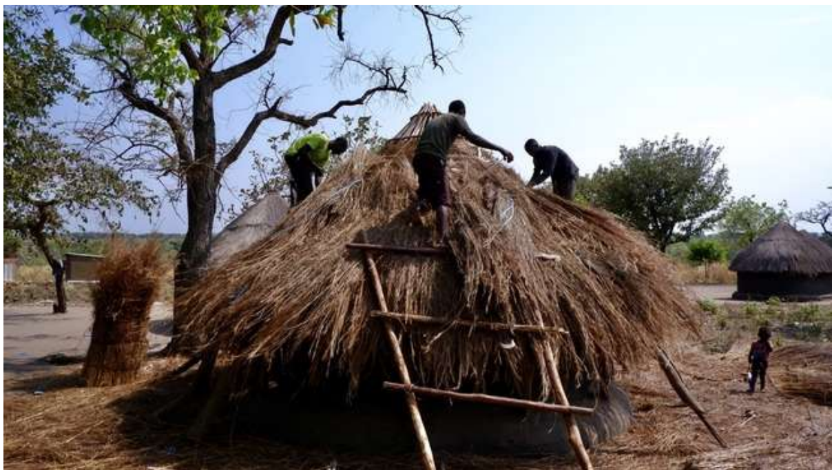
Figure 26. Maintaining a grass roof.
