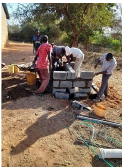
Image 10: Well building demonstration.
