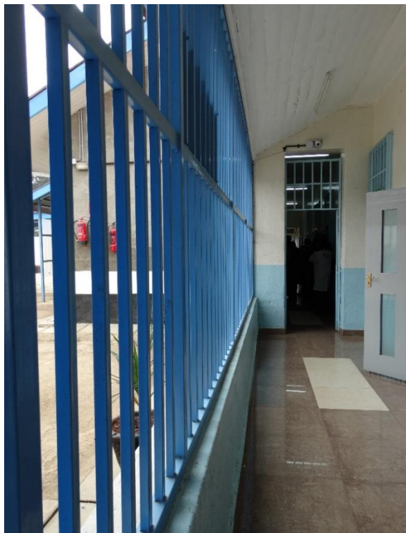
Figure 5.7 Hallway with security bars in the enclosed building of the MAT clinic (EC)
