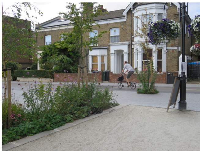
Fig. 3. Example of a modal filter, Walthamstow neighbourhood (source: Rachel Aldred).
