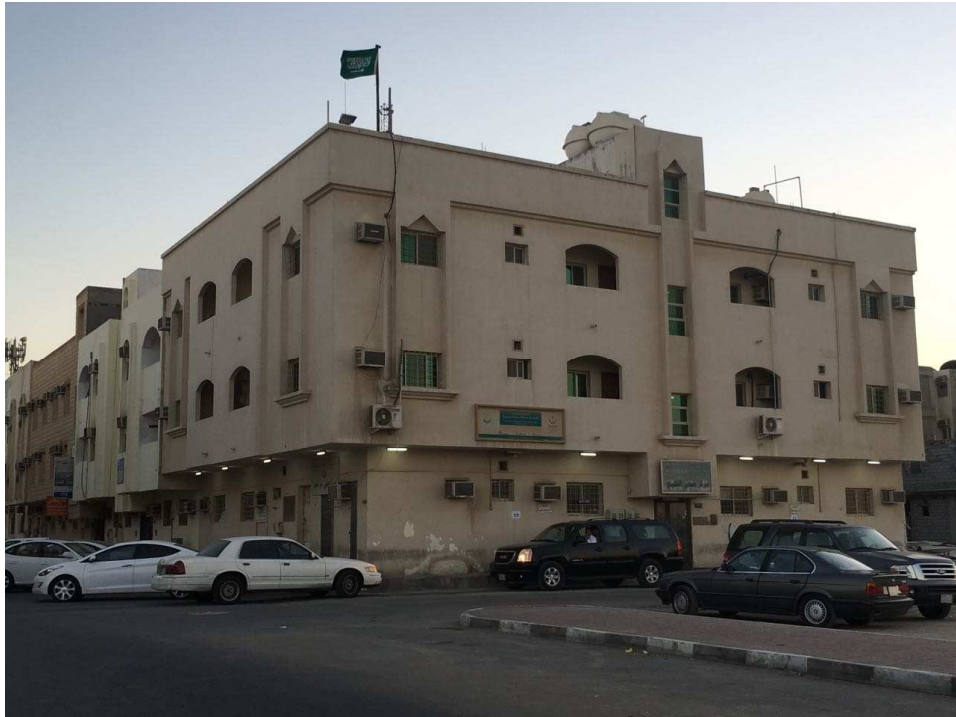
Figure 5: Al-khaleej Primary Health Care Centre
