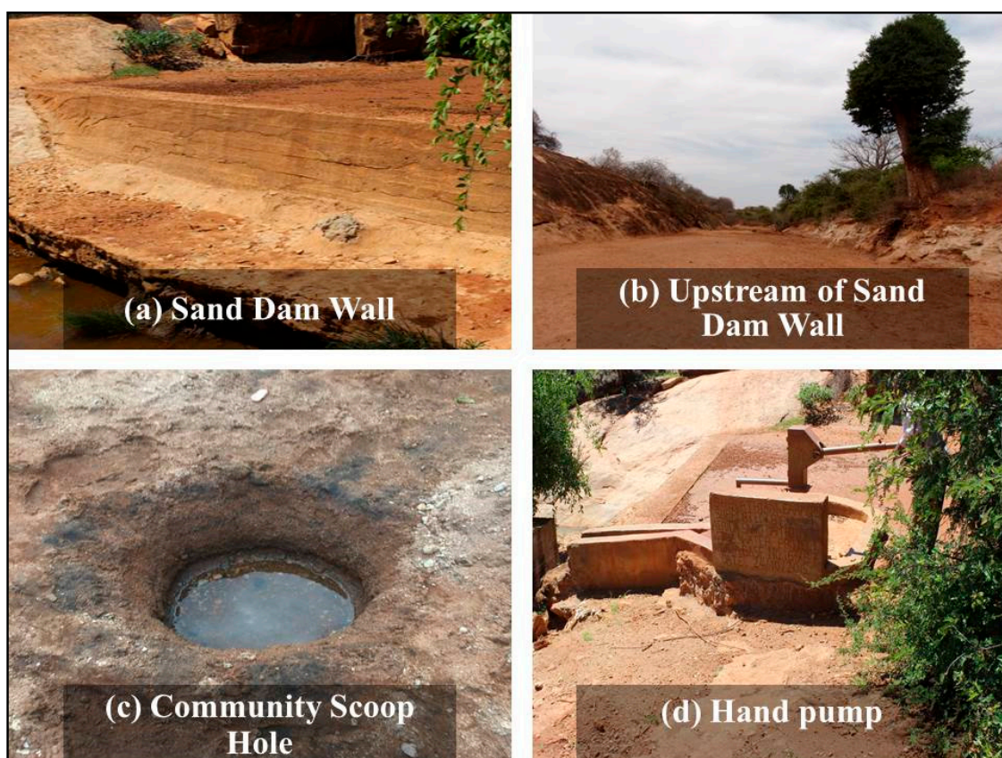
Figure 1. The sand dams and their water abstraction methods.
