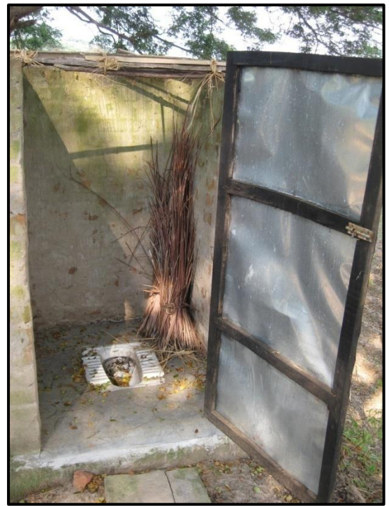
Figure 6. An unused completed latrine in Sankhatira village
