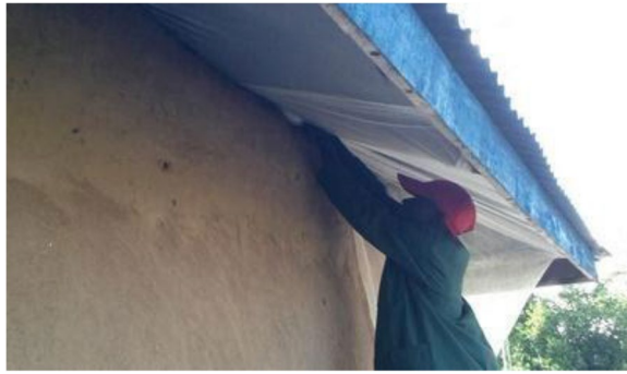
Fig. 1 ITENs being installed. The net is provided on a roll and takes only thirty min to install, but lasts more than 4 years in Kenya
