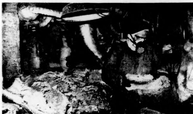
FIGURE 2.8: Asbestos debris in a boiler room.
