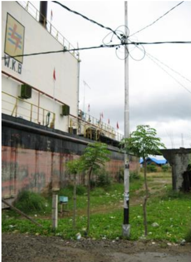
Power barge washed 5km inland into an Aceh village, 2004 Photo L Reynolds
