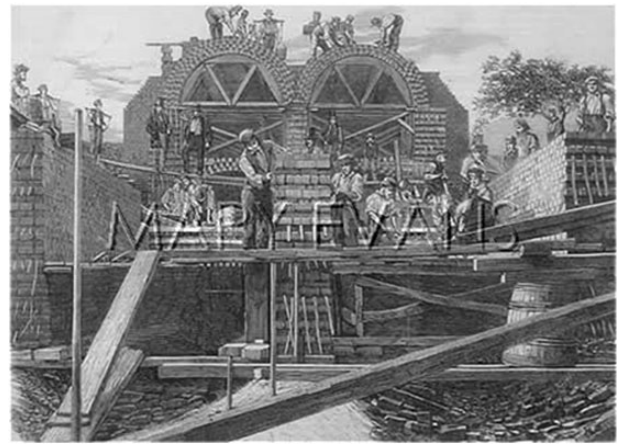
Fig. 1 London Sewer Construction in Bow, 1859. Copyright Illustrated London News/Mary Evans Picture Library, ref 10010475. The public health service in its Victorian phase is associated with major capital projects, authorized and resourced by elected councils. In Thomas McKeown's famous account of the modern rise of population, he calculated that 33% of the mortality decline between 1848/54 and 1901 was attributable to water-borne diseases amenable to such interventions. 8
