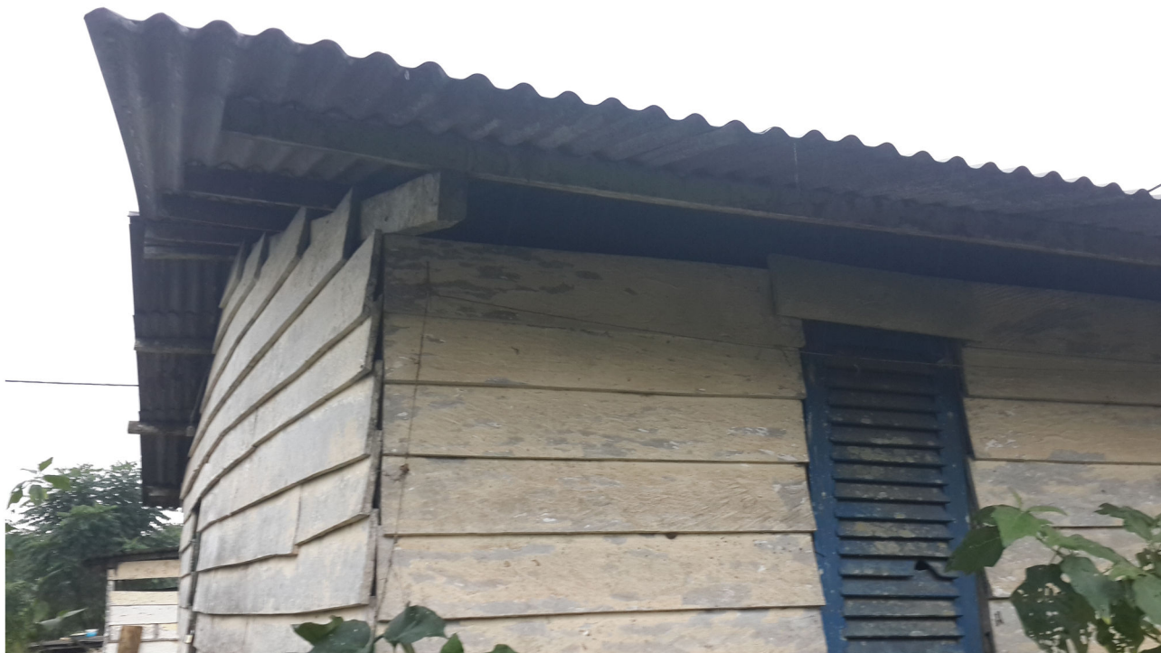
Figure 1. An example of a house on Bioko with wooden walls and open eaves.
